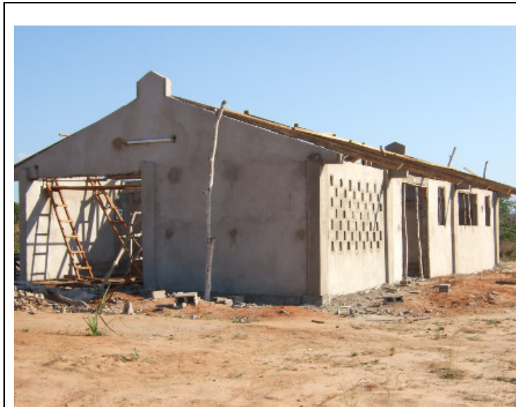
The nearly completed workshop (photo November 2008).
