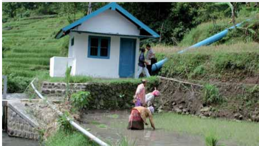
This picture shows the turbine house of a micro hydro power facility in Indonesia. EnDev activities in Indonesia concentrate on “Micro Hydro Power for Sustainable Economic Development” for institutional, domestic and productive use. The Mini Hydro Power Project (MHPP) in Indonesia follows a commercial approach ensuring a continuous sustainable growth of the MHP market.
