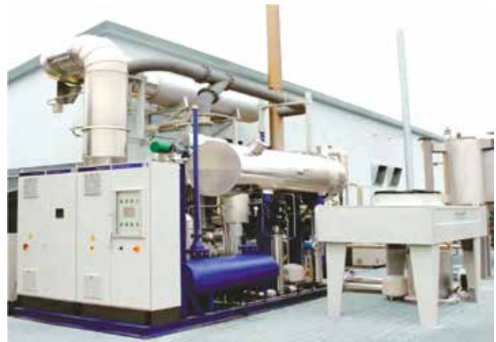
Figure-1 ORC system in Groß-Gerau
