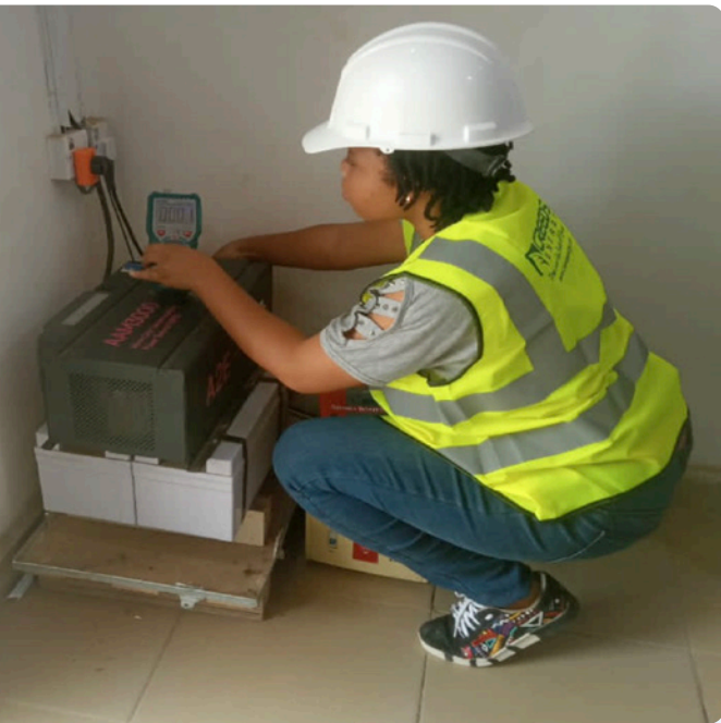
Figure 3. Testing and commissioning of system (Source: CREEDS)
