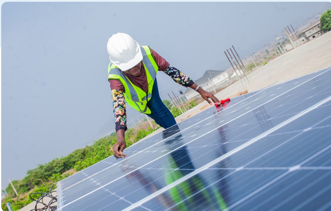
Figure 1. Installation of LiteDey system (Source: CREEDS)
