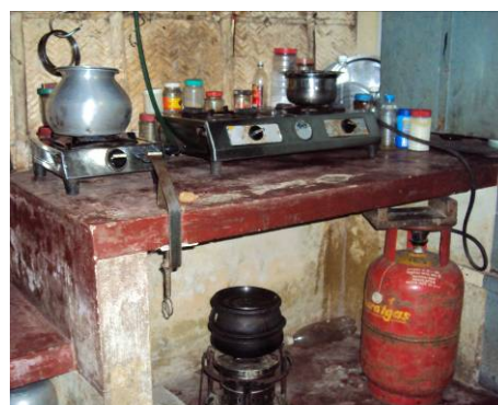
Figure 32: Typical kitchen in Kumbalanghi with the single biogas stove and the double LPG stove.
