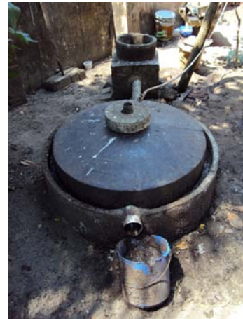
Figure 19: On the left (a): Face to face interviews. In the middle (b): 2m 3 toilet linked biogas plant. On the right(c): 1m 3 ordinary biogas plant.
