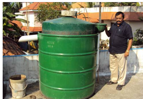
Figure 6: 1m 3 fibreglass reinforced plastic plant for the treatment of kitchen waste.
