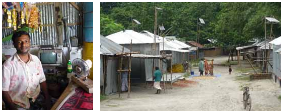
Figure 1 – Solar Home System units and panels, Source: SLE-Team
