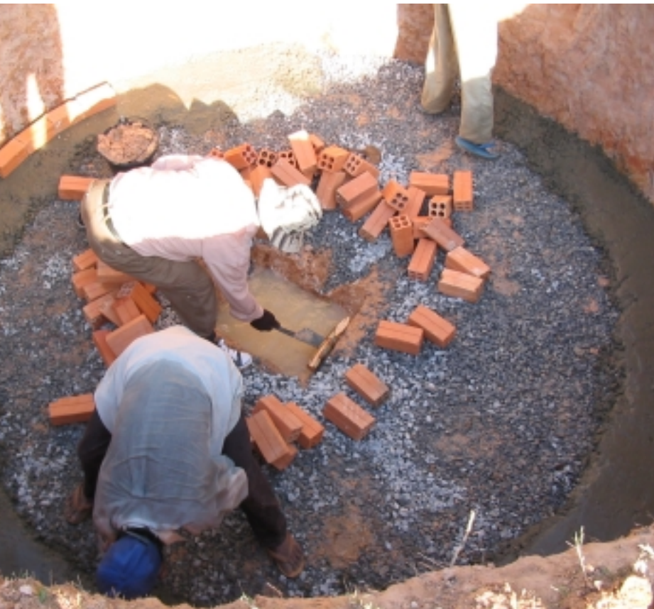
Figure 11 Constructing the Base
