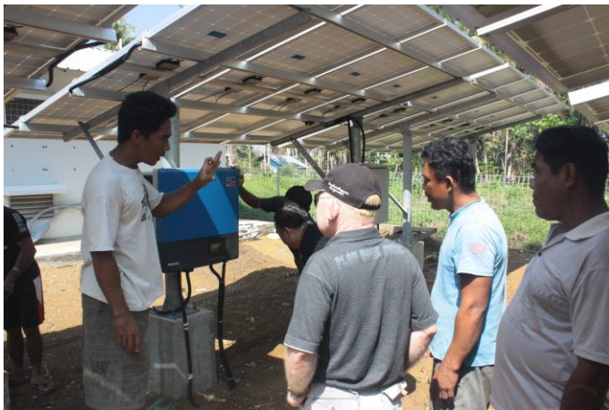
Figure 25 – The operator explained on how a Solar Power Plant (PLTS) works
