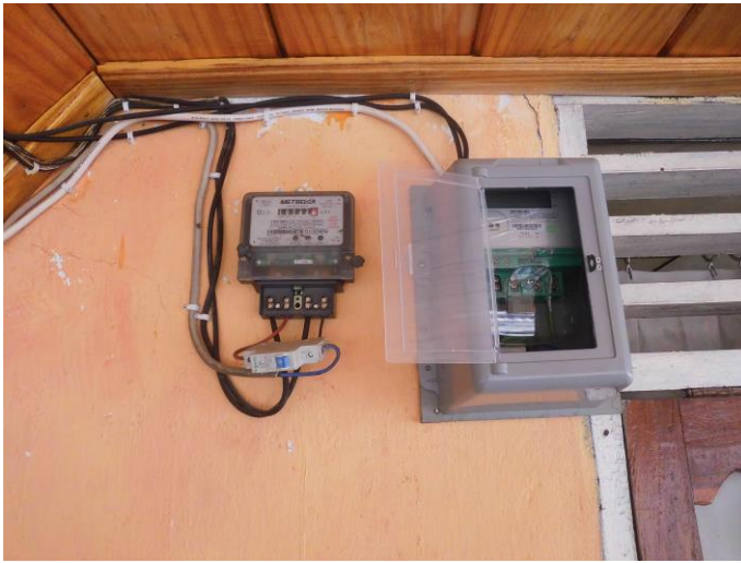
Figure 24 – The energy limiter at Solar Power Plant (PLTS) electricity receiving houses in West Lamdesar, Larat Island
