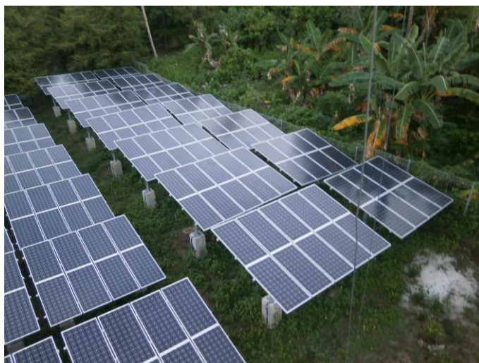
Figure 2 – The 50 kWp capacity of Solar Power Plant (PLTS) in Kawaluso Island provides electricity for 153 families
