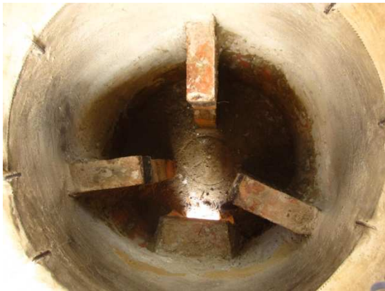
Pot rest made out of fired bricks in a round stove construction
