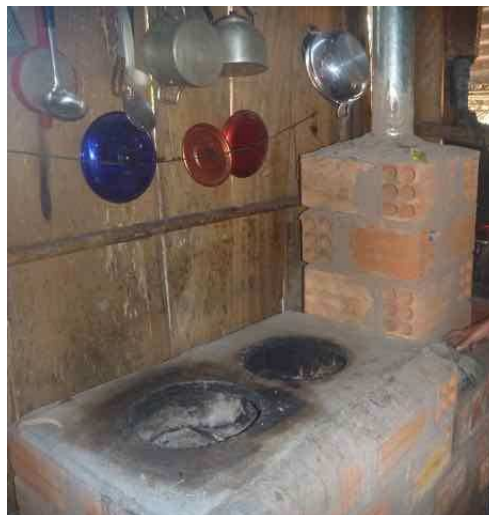
Metal chimney, insulated with bricks at lower part
