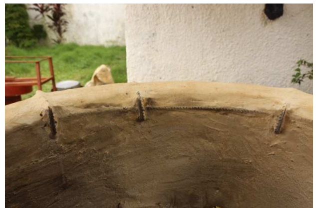
Close view of the metal ring with distance holders, sitting on top of the round structure of the stove, covered by plaster for heat protection
