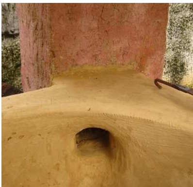
Entrance of the chimney is at the highest point to maximize the area where the pot is in touch with the hot gases
