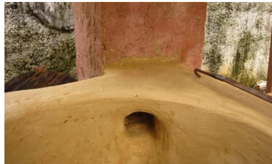
Entrance of the chimney is at the highest point to maximize the area where the pot is in touch with the hot gases
