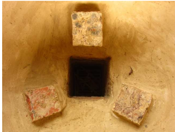
Pot rest made out of fired bricks, located at plastered "bowl" for pot
