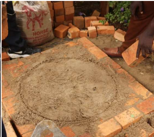
brick layer as foundation
