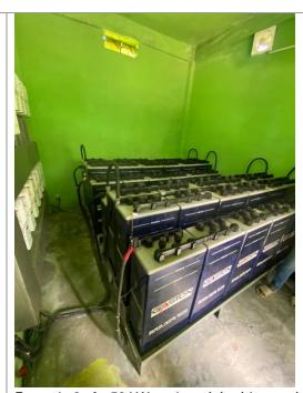
Example 2 of a 50 kWp solar mini-grid powering a health clinic, ~100 solar street lights and 180 households with 2 lights and a charging port. Batteries pictured are lead acid based on local market availability and recyclability.
