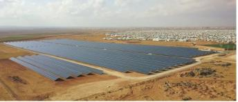
Example 1 of a grid-tied solar mini-grid, providing power to Zaatari refugee camp, with a capacity of 12.9 MW. In refugee settings, it's likely the capacity would be smaller.
