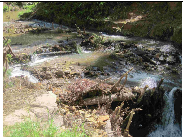
Photo 2: Same weir in Oct 10
