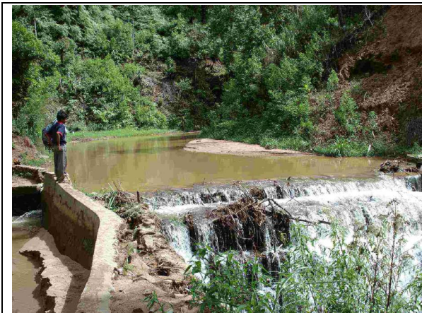
Photo 1: Weir in Minangga in Nov 07
