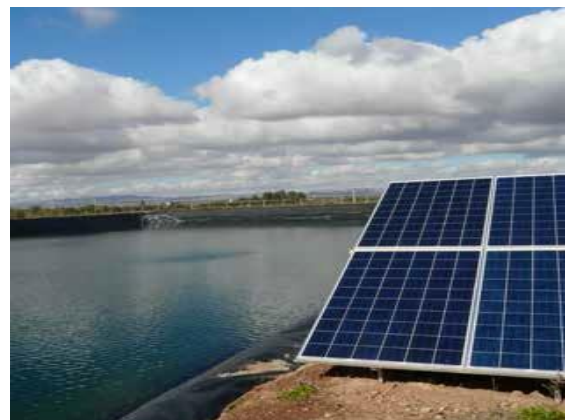
Open plastic foil-lined reservoir
