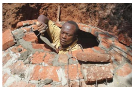
Domestic fixed-dome biogas system being constructed in Tanzania www.biogas-tanzania.org
