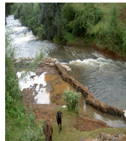
Existing Canal of gobocho II
