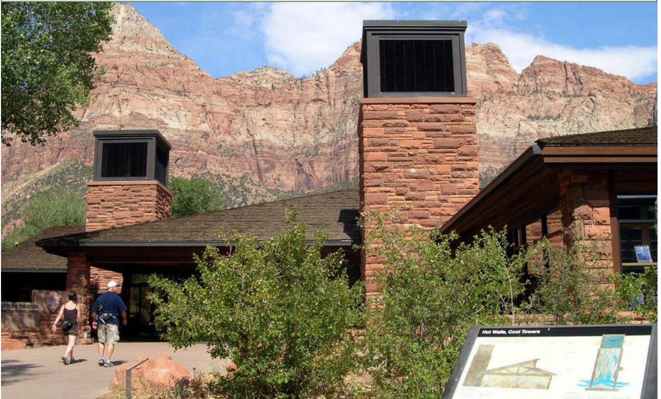
Figure 42: Evaporative cooling tower. Source: Picture by Tim Vo ©Creative Commons 14
