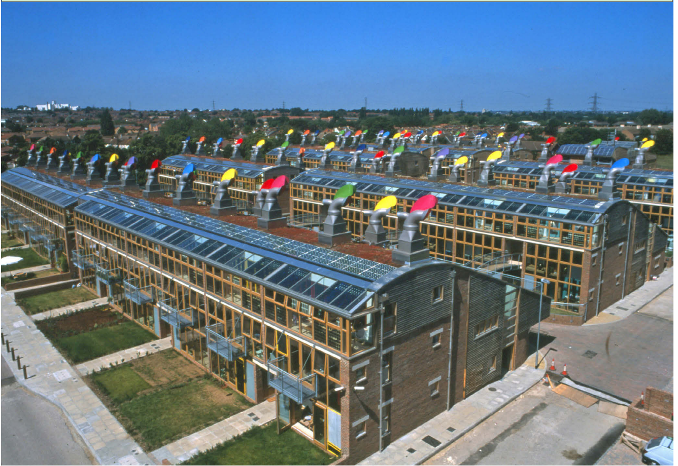
Figure 14: BedZED community development (courtesy of Wikimedia commons) © Arup
