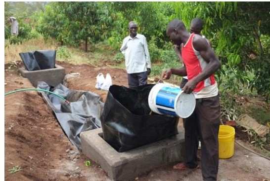
Training course for biogas construction
