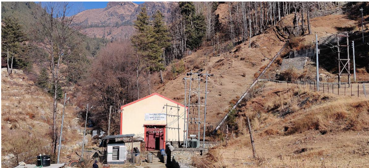
Figure 2-5: Powerhouse of 200 kW Ghughuti MHP
