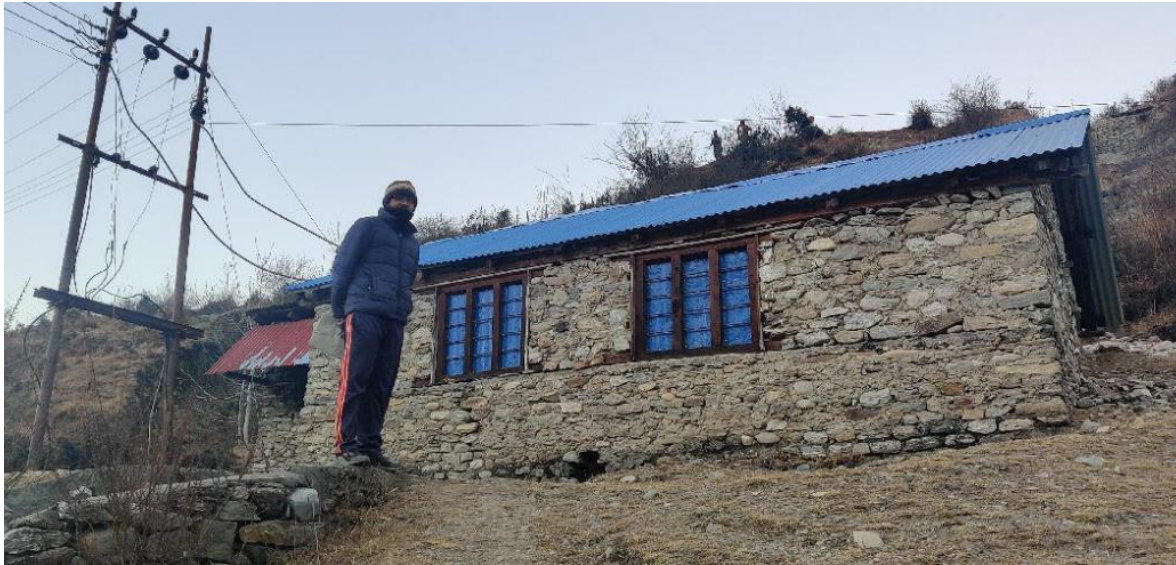
Figure 2-2: Powerhouse of Triveni MHP
