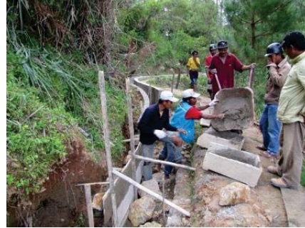
Photo 19: Civil construction, West Sulawesi
