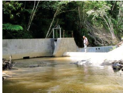
Photo 22: Inspection, Mesakada, West Sulawesi
