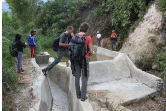
Photo 21: Testing of civil works, Sulawesi
