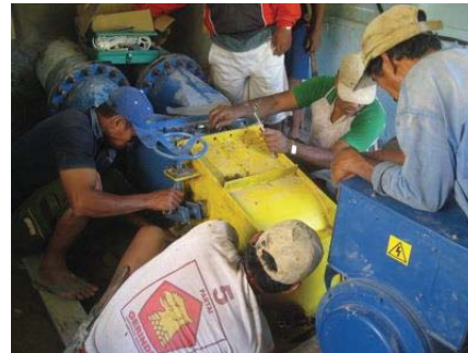
Photo 20: Turbine installation
