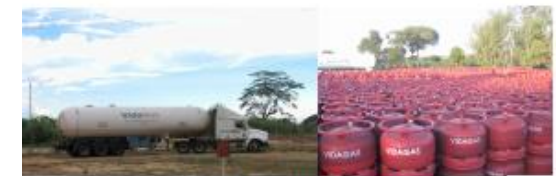
VidaGas Transporter & Filling Plant
