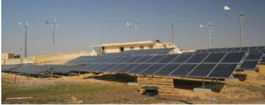
Wind-Solar-Diesel-Battery System, Egypt
