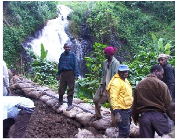
The entire penstock was supported by soil bags wherever possible and covered to prevent damage by sunlight.
