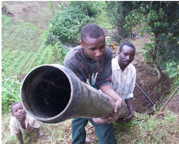
Sockets enable the 6m pipe lengths to be fitted together. An 'O' ring fits in the socket recess and provides a pressure tight seal.
