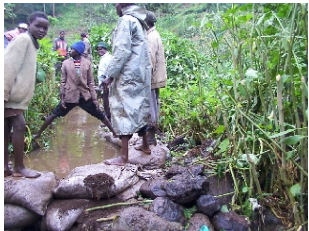
Boulders have been used to form a deep pool around the intake. Soil bags seal the gaps.
