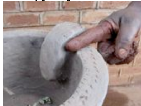
potrest height should be 1.5 cm (one finger) and flat on the top to prevent pots from wobbling
