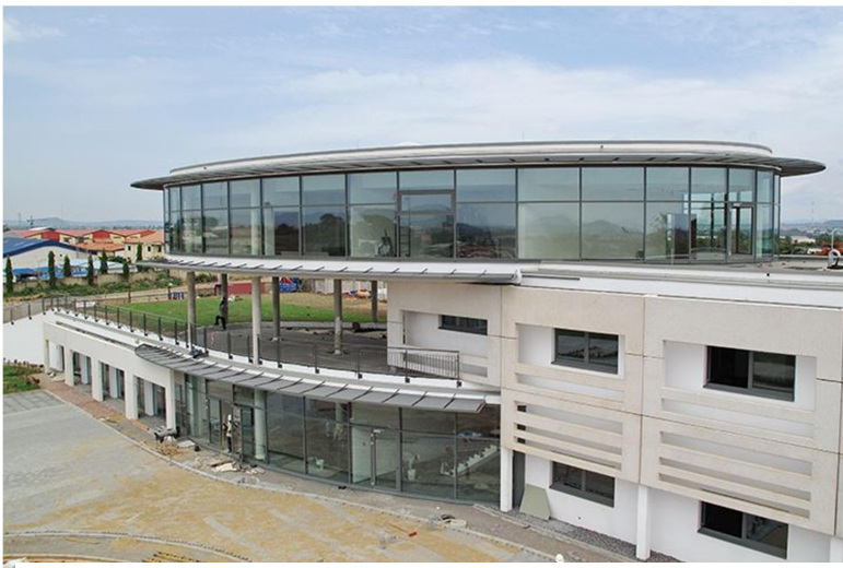
Figure 3.21: Front view of the PrimeTech head office
