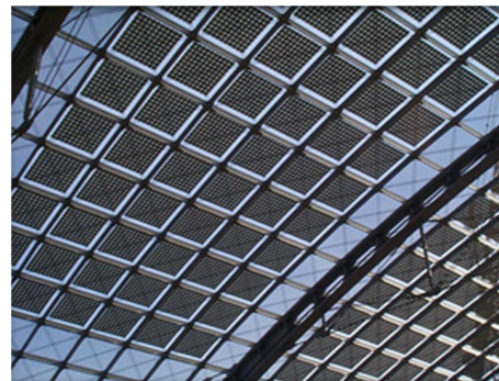
Figure 4.6: Roof integration of transparent PV modules .Central railway station, Ber-
