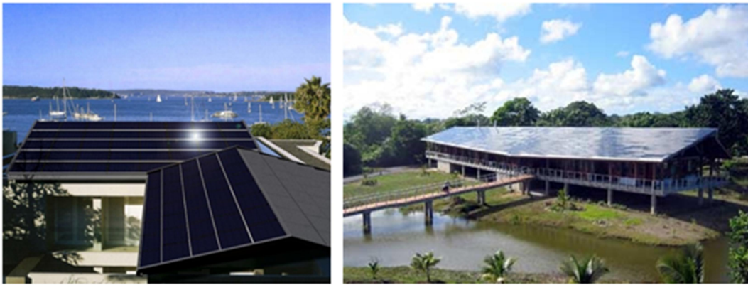
Figure 4.4: Roof-integrated PV panels – Source: images.google.com
