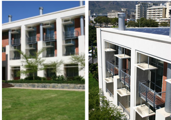
Figure 3.25: Combined shading and daylighting devices in north facade of BP Headquarter in Cape Town: Light shelves, roof overhangs, and balconies.
