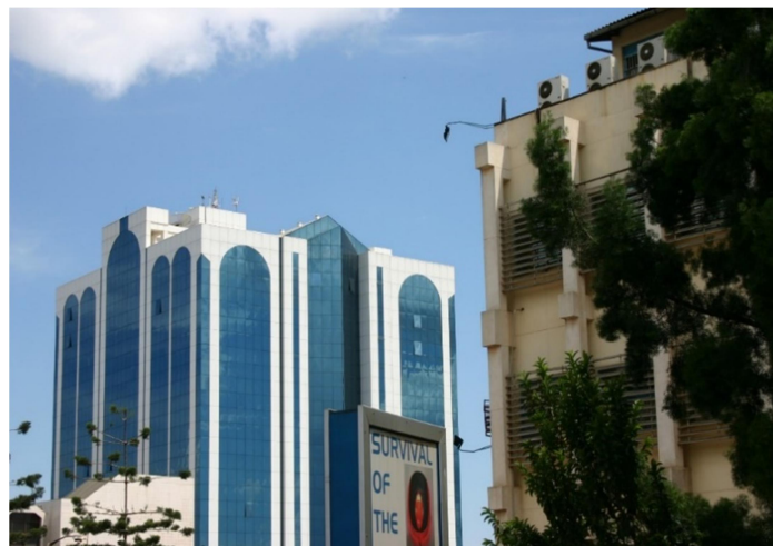
Figure 3.26: Exterior shading by horizontal aluminium lamella (front) and reflective coating of glass (background, workers house) Kampala, Uganda
