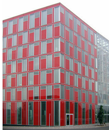
Figure 3.61: Capricorn office building in Düsseldorf, Germany, with facade integrated air conditioning. The complete technology for ventilation, heating, cooling and heat recovery is positioned in the 20 cm deep façade – Source: Architects Gattermann und Schossig
