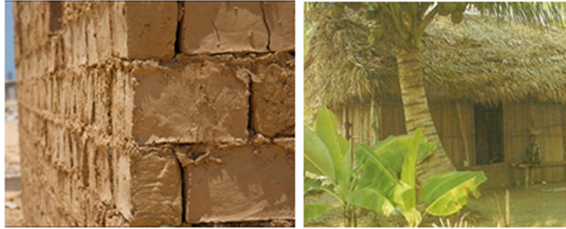
Figure 3.14: Mud bricks, perfect for their thermal inertia (left), house in south Nigeria with light walls and a palm roof, to enhance inner ventilation (right) – Sources: news.bbc.co.uk , images.delcampe.com
