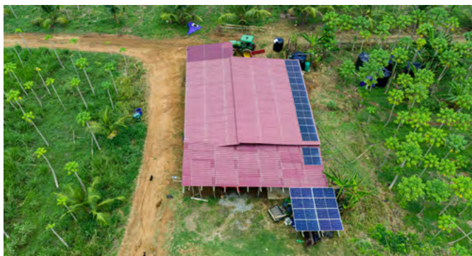
Picture 1: PV Pump Installation
