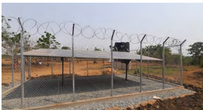
Picture 2: Solar Pump System
