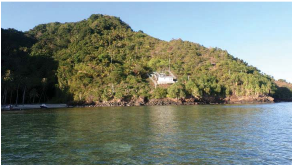
This PVVP installation on a small remote rocky island demonstrates the installation challenges faced by contractors.
