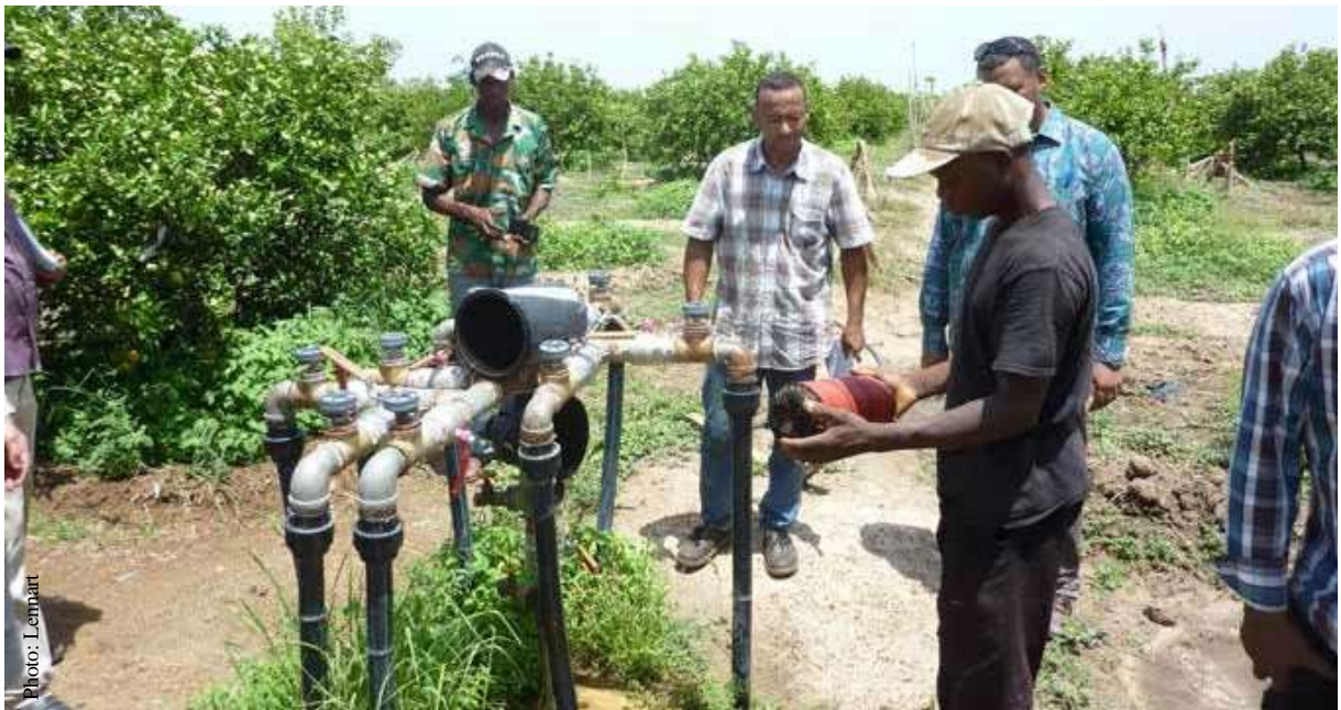
Irrigation head with a disc filter and multiple valves that guide the water to different sections of the irrigation system (Source: Lennart Woltering).
