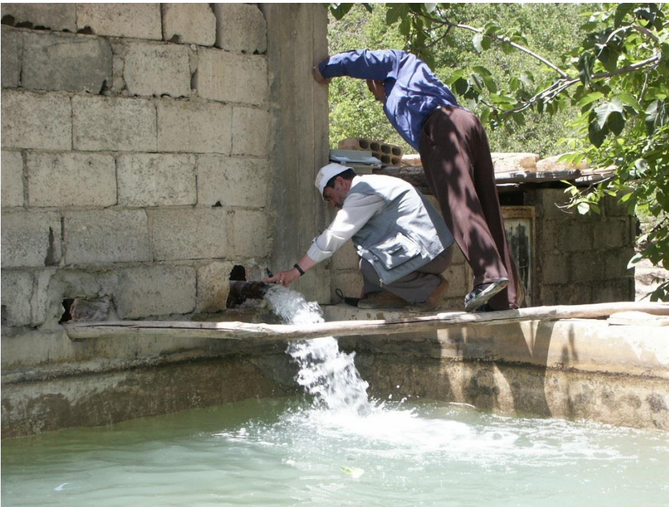
Groundwater pumping and short-term storage
