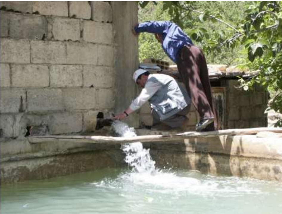
Groundwater pumping and short-term storage
