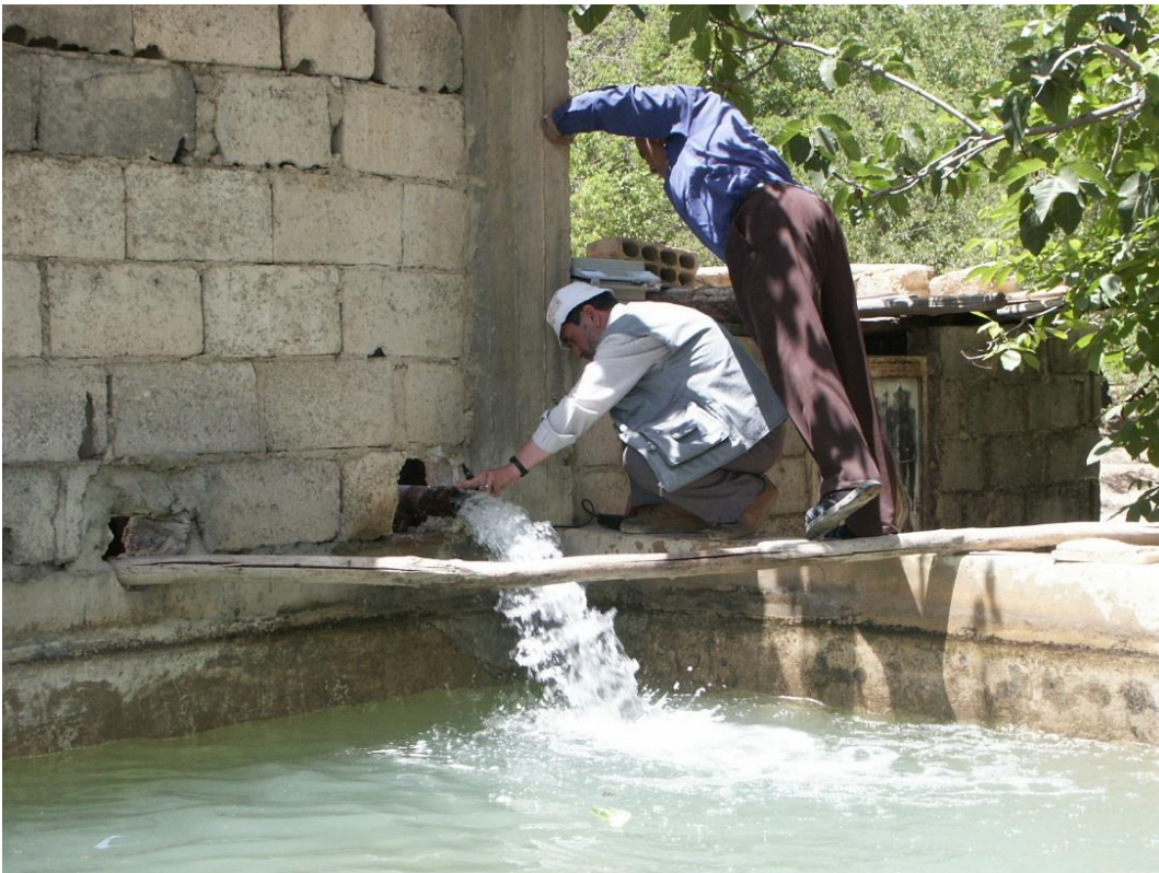
Groundwater pumping and short-term storage
