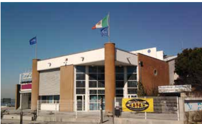
The Bibione Mare harbor building
