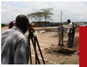
Land survey at Talek Power location. A minigrid developer must have environmental clearance in the form of an ESIA licence issued by NEMA before starting construction.
