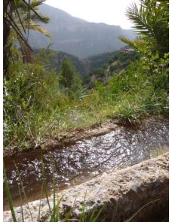
Concrete irrigation canal
