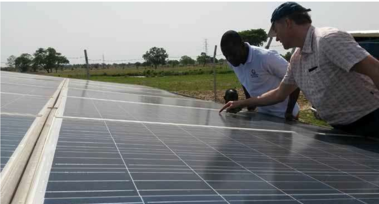
Visual check of the solar panels
