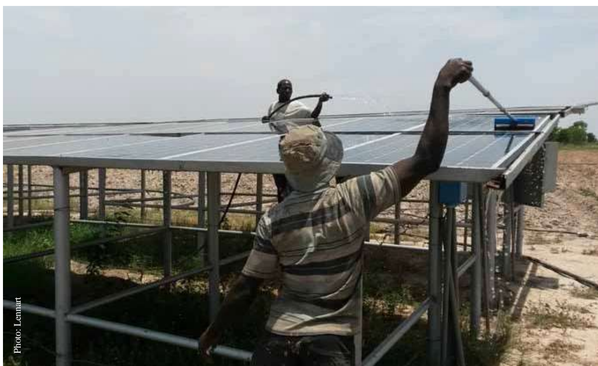
Cleaning of solar panels in Ghana as a routine maintenance activity
