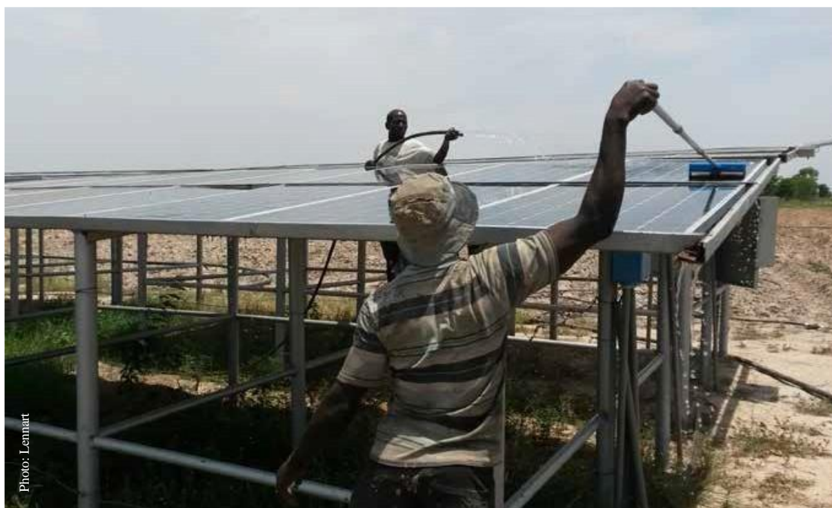
Cleaning of solar panels in Ghana as a routine maintenance activity (Source: Lennart Woltering)
