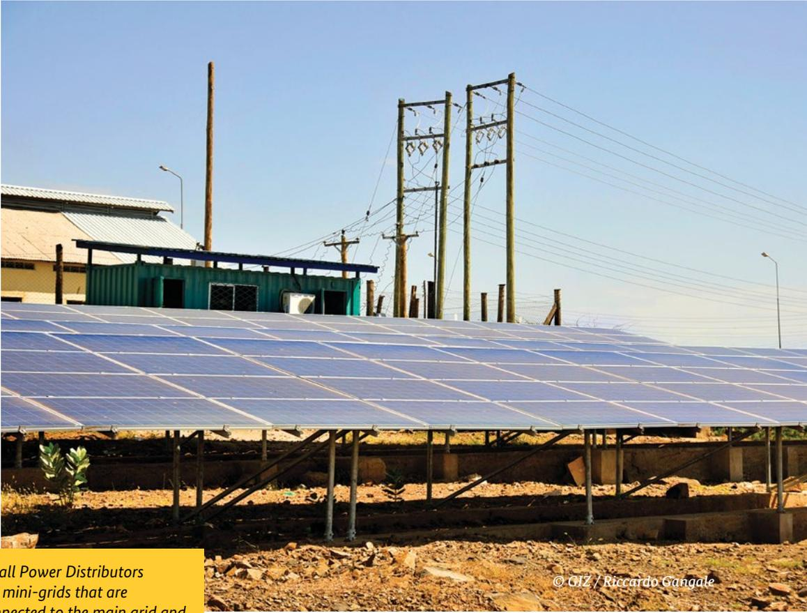
*Small Power Distributors are mini-grids that are connected to the main grid and complement grid-electricity with a solar plant*
