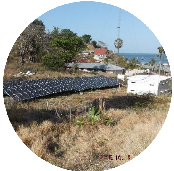
A 30 kWp PV micro-grid in Luang Barat Village, Maluku Barat Daya District providing electricity for 145 households and 8 public facilities.
