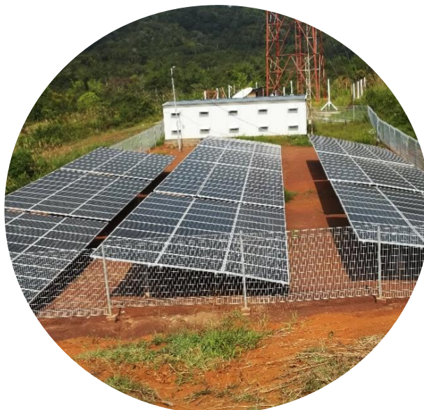
A 50 kWp PV micro-grid in Long Layu Village, Nunukan District, Kalimantan Utara built by KESDM under 2014 budget (Source: EnDev ID, GIZ)
