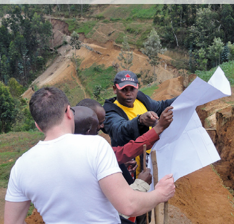
Ruanda: EnDev consultant and project developers discuss at the building site of Mazimeru Micro Hydro Plant.
