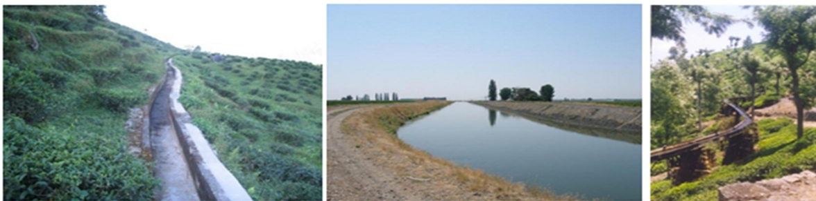
Figure 3.114: Examples of masonry: Lined (left), earthen (middle) and wooden (right) channels
