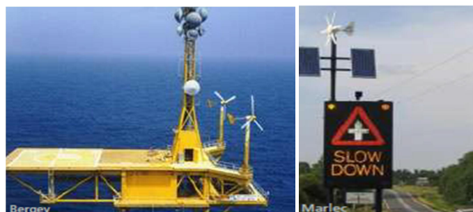
Figure 3.157: Remote power supply for meteorological platform at sea (left), traffic signal (right)
