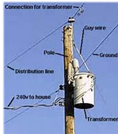
Figure 4.10: Single-phase transformer on a pole
