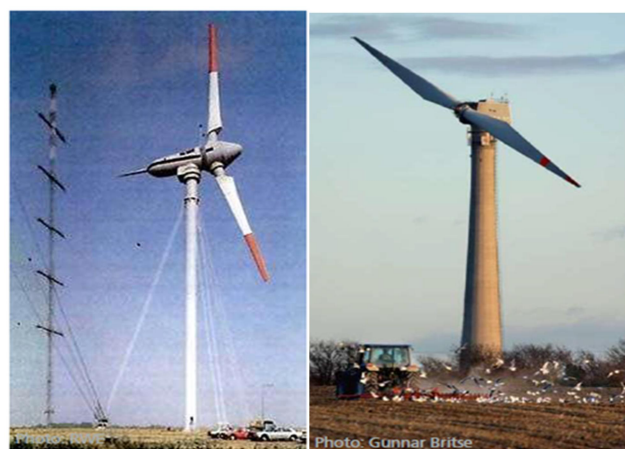
Figure 3.143: Dual-blade wind turbines of 3 MW in Brunsbüttel, Germany, 1983 (left) and 2 MW in Näsud-den, Sweden, 1983
