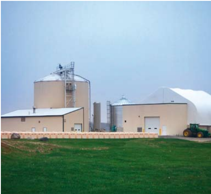
Biogas plant for liquid cattle manure in Ravenna, Michigan, USA
