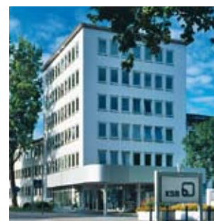
KSB administration building
