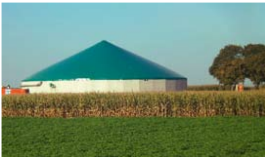
Air-inflated structures and silo covers of the feedstuff drying Kaufbeuren biogas plant
