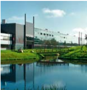
EISENMANN Holzgerlingen technology park and assembly centre
