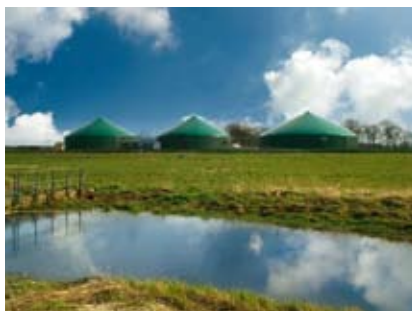
Ardorf natural gas
