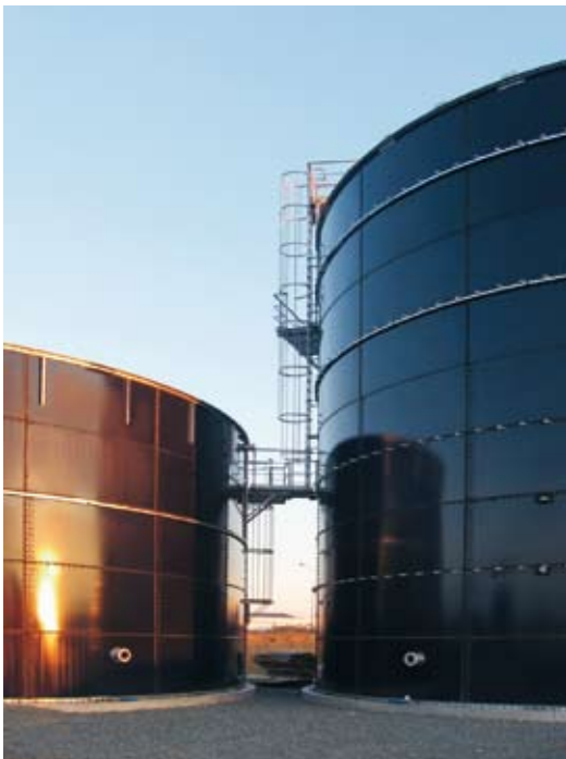
Schwarting biogas plant in France
