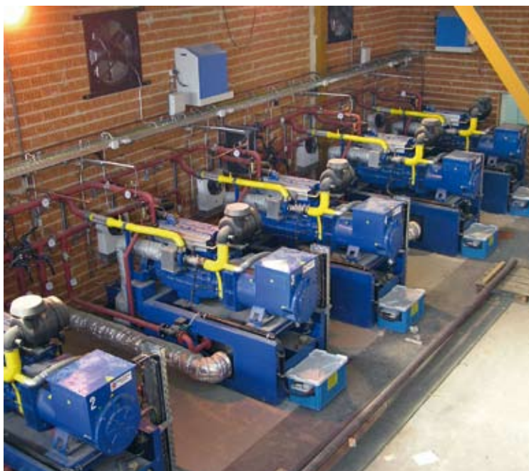
Finished system with six pilot-injection cogeneration units
