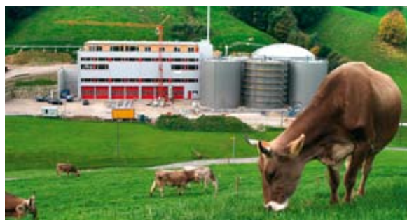
Production residue disposal plant
