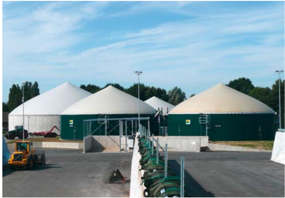
Biogas plant at Kirchlengern
