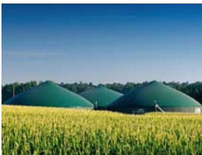
A typical MT-ENERGIE biogas digester system
