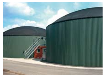
PlanET biogas plant
