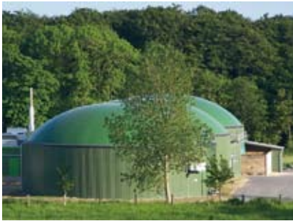
Biogas plant in Wittkiel
