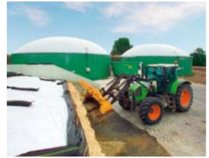
Individual biogas plant with fermenters made from reinforced concrete
