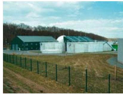
Municipal biogas plant in Germany: 795 kW el Input: 35,000 tons of farming biomass Hygienisation of the biogas substrate
