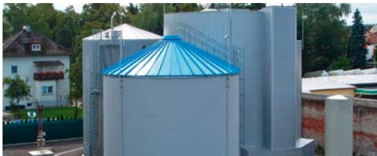
Plant for anaerobic whey-waste water treatment
