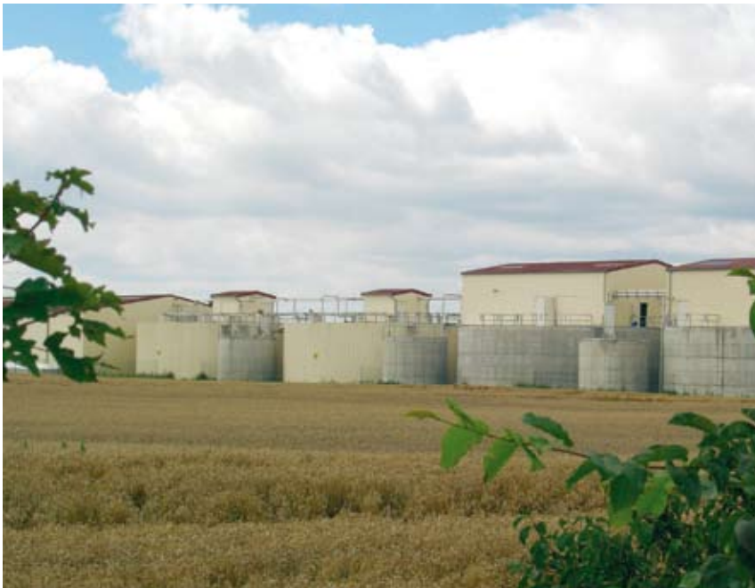
Hammlar biogas plant for the fermentation of production residues from a herbal drying facility
