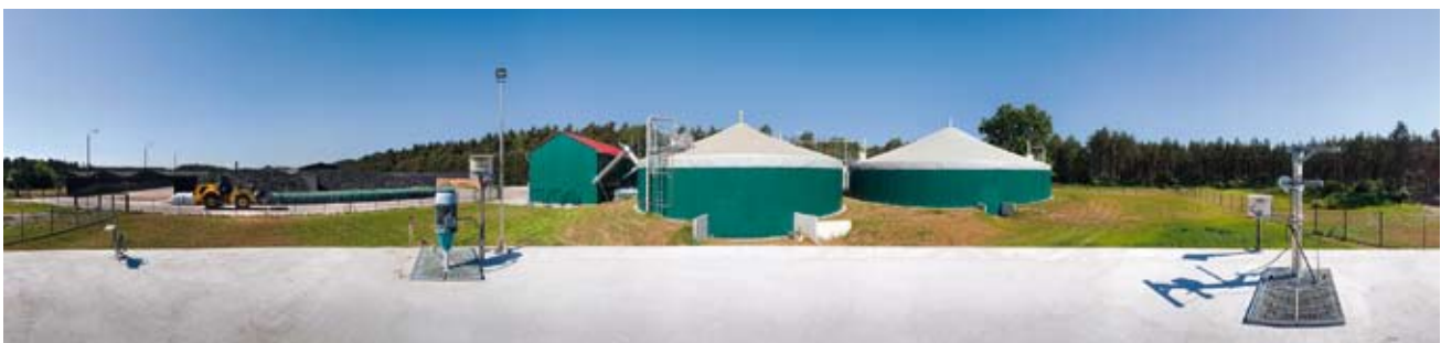
Biogas Plant Gut Borken (740 kW)
