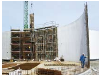
Postfermenter of the biogas plant under construction
