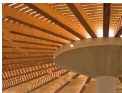
Wooden ceiling of a fermenter under construction
