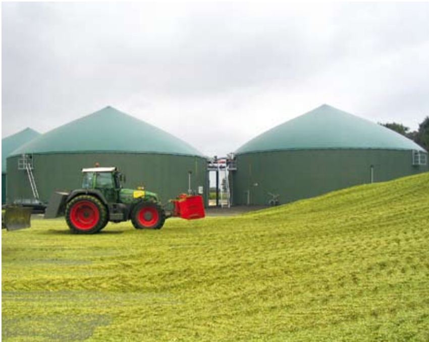
Wetschen biogas plant
