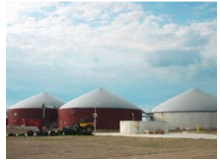
Neukirchen biogas plant
