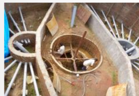
biogasreactor in the center of the building
