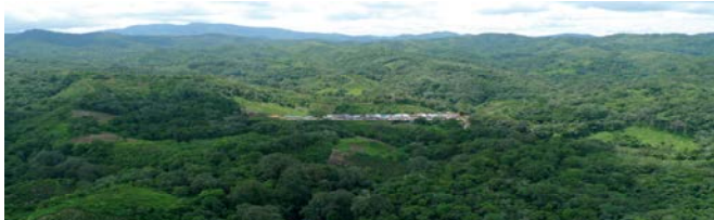
Photo: Long house in the outback of Malaysia powered by PV-MINI Grid
