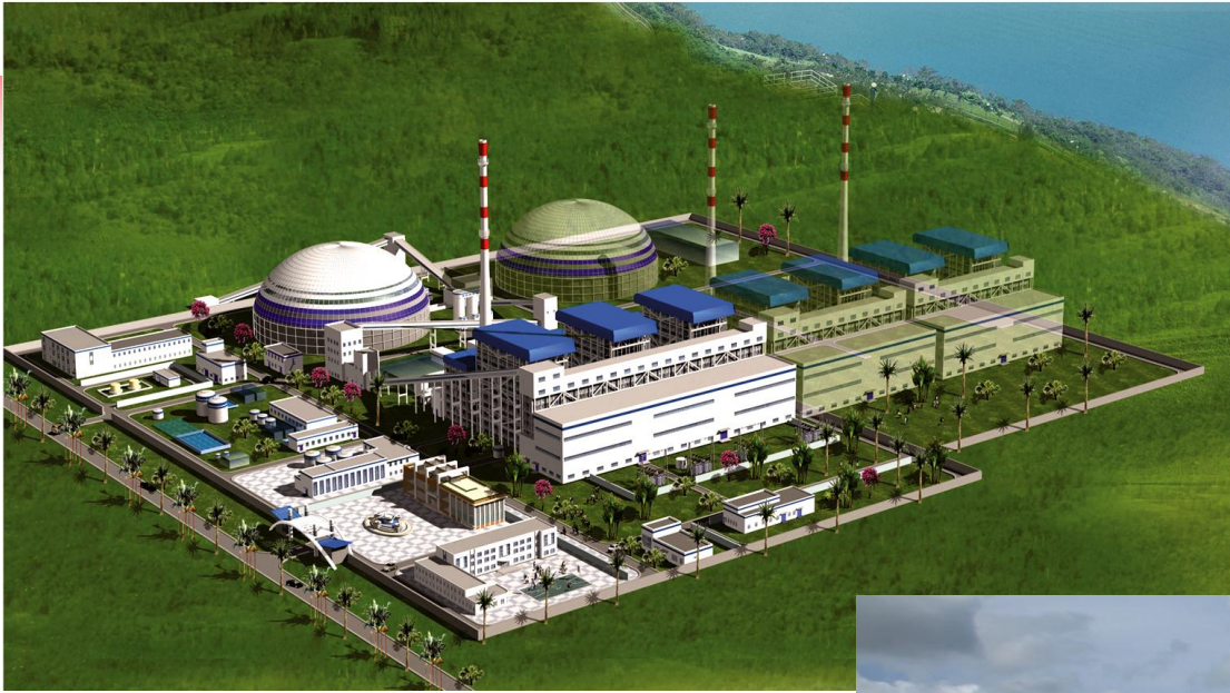
Sihanoukville 7 × 135MW coal-fired power plant aerial view
