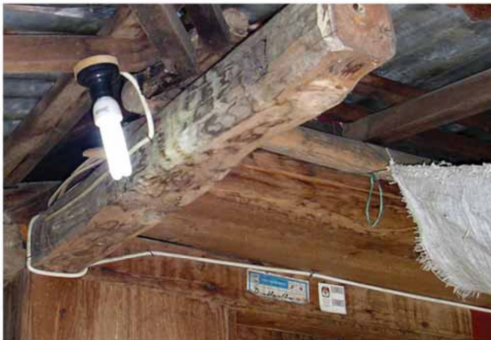
Lamp installation - good
