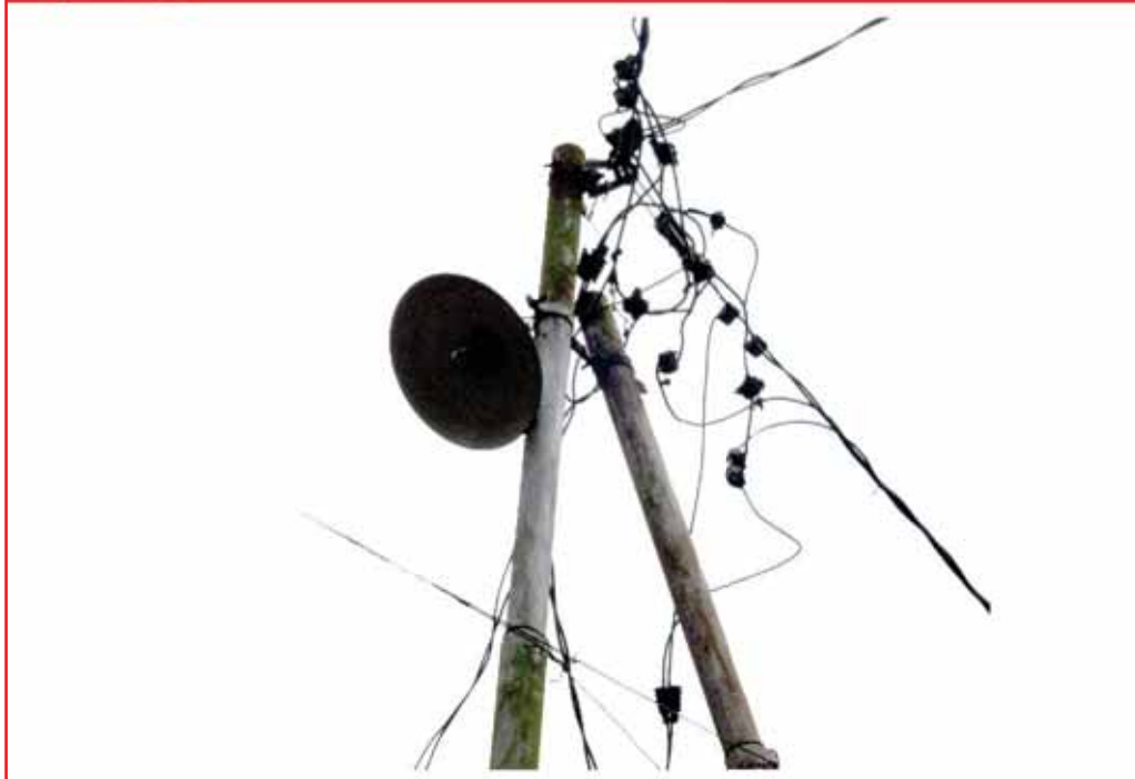
Bad example of a wiring connection
