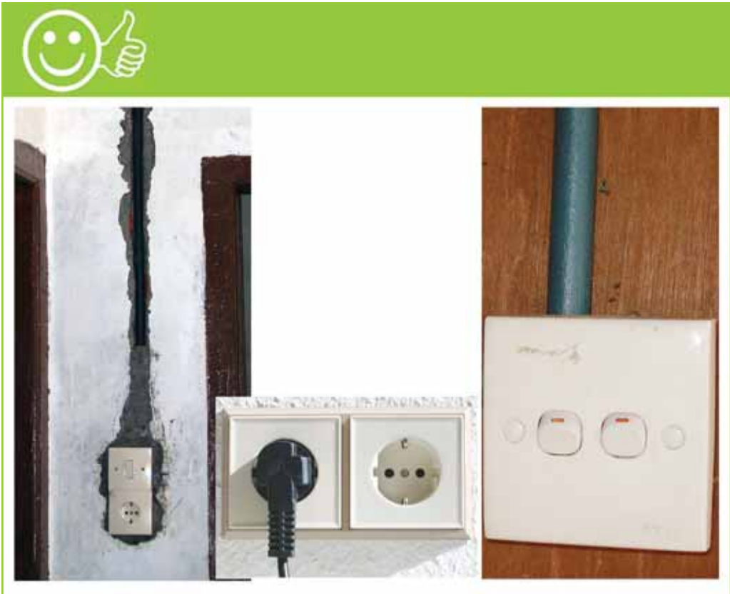
Sockets, plugs and switches - good
