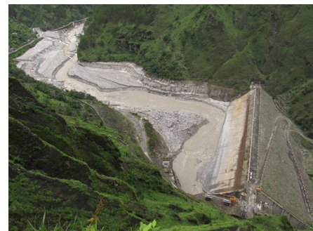
Figure 3.22: Dhauliganga dam, India
