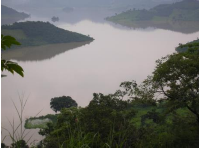
Figure 1.20: Example of large storage
