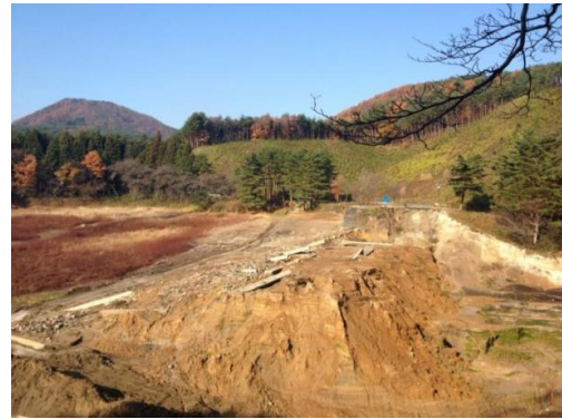
Figure 3.17: Fujinuma dam in Japan failed due to an earthquake
