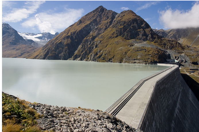
Figure 3.14: The Grande Dixence Dam (Switzerland) is the world's highest concrete gravity dam (285 metres)
