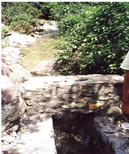
Figure 3.7: Intake top wall
