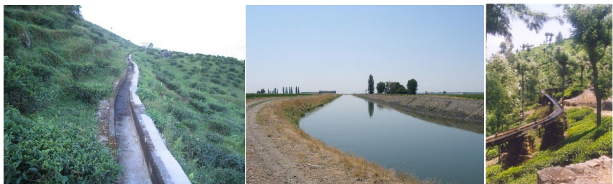
Figure 1.7: Examples of masonry: Lined (left), earthen (middle) and wooden (right) channels
