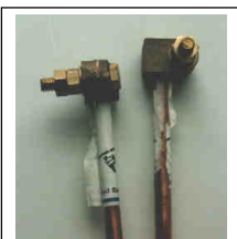
Figure 9-3 Installation of a copper-plate earth electrode. Multiple earth cables have been soldered in place to reduce the resistance and increase the reliability. (Nepal)
