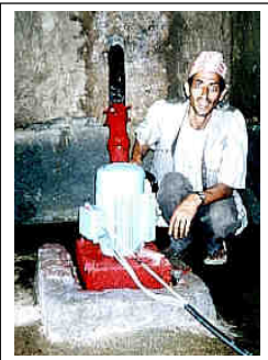
Figure 8-1 The 'Peltric Set' has provided many rural villages with an economical electricity supply in Nepal
