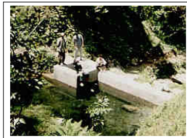
Figure 10-4 A concrete weir can be used to form a small reservoir (Nepal).
