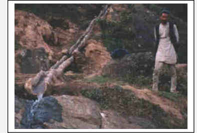
Figure 10-8 A wooden aqueduct can be used to transport water in the canal across uneven ground
