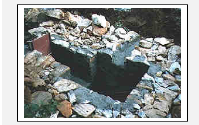
Figure 10-16 The flow of water into the forebay is controlled by a sluice gate. An overflow is cut into the wall on the downhill side so that excess water is returned to the stream without undermining the masonry. A flushing pipe, sealed with a wooden bung has been incorporated at the lowest part of the tank.
