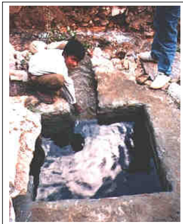
Figure 10-12 A small forebay is suitable where flow is sufficient throughout the year
