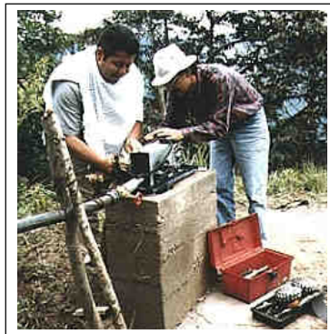
Figure 8-2 A Colombian manufacturer (right) installs a DC pico hydro system.
