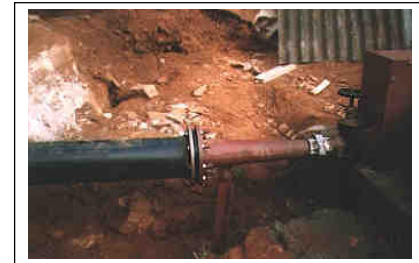
Figure 11-10 Penstock connection using flanges
