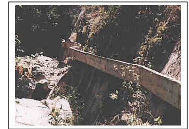
Figure 10-6 Canal installed in a difficult location supplying a small hydro scheme for local electrification (Peru)
