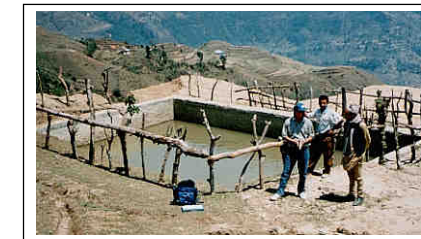
Figure 10-17 A small reservoir provides low-cost energy storage which can be useful during the dry season. (Sankhuwa Sava, Eastern Nepal)
