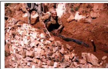
Figure 11-6 The supports must be suitably reinforced before filling the pipe.
