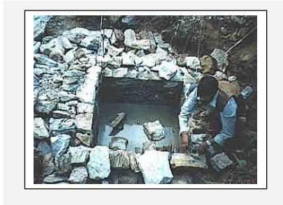
Figure 10-15 Construction of stone forebay (Kushadevi, Nepal)
