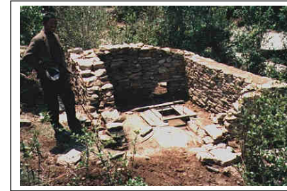
Figure 12-3 Power house under construction, Nepal
