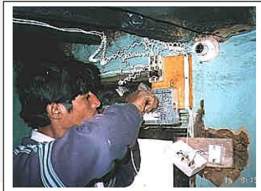
Figure 15-1 Installation of domestic wiring circuit (Nepal)
