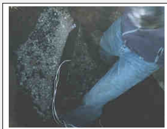
Figure 9-3 Installation of a copper-plate earth electrode. Multiple earth cables have been soldered in place to reduce the resistance and increase the reliability. (Nepal)
