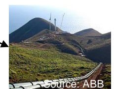
El Hierro, Spain Hydro (pump. storage), wind, diesel, control sys.
