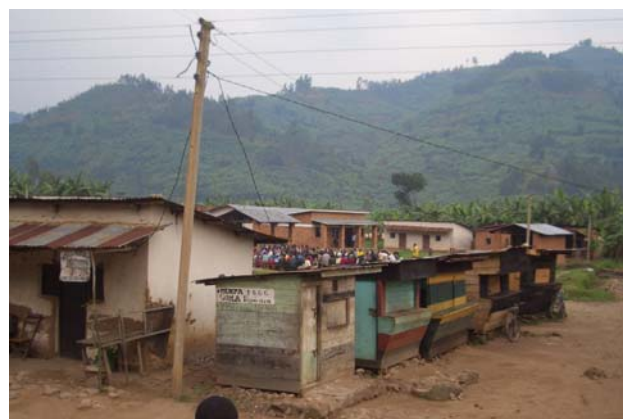
Photo 7: Electricity Grid at Nyamyotsi [NI c ]
