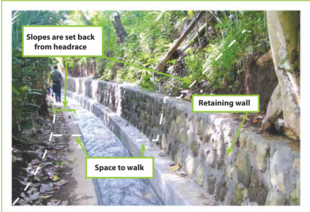
Retaining wall stabilizes the toe of the slope
