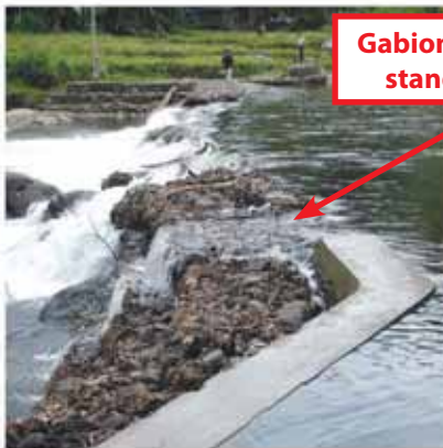
Examples of unsuitable dam materials
