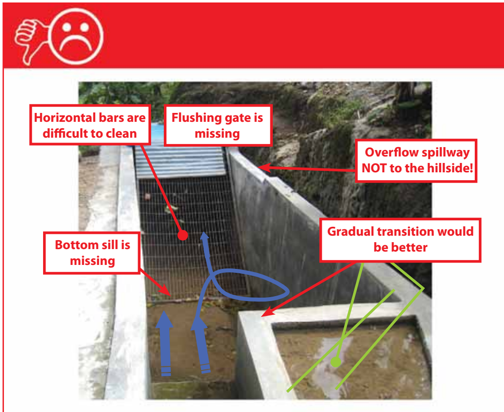
Forebay without sedimentation
