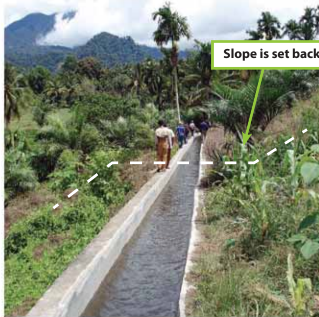
Headrace channel is free of vegetation
