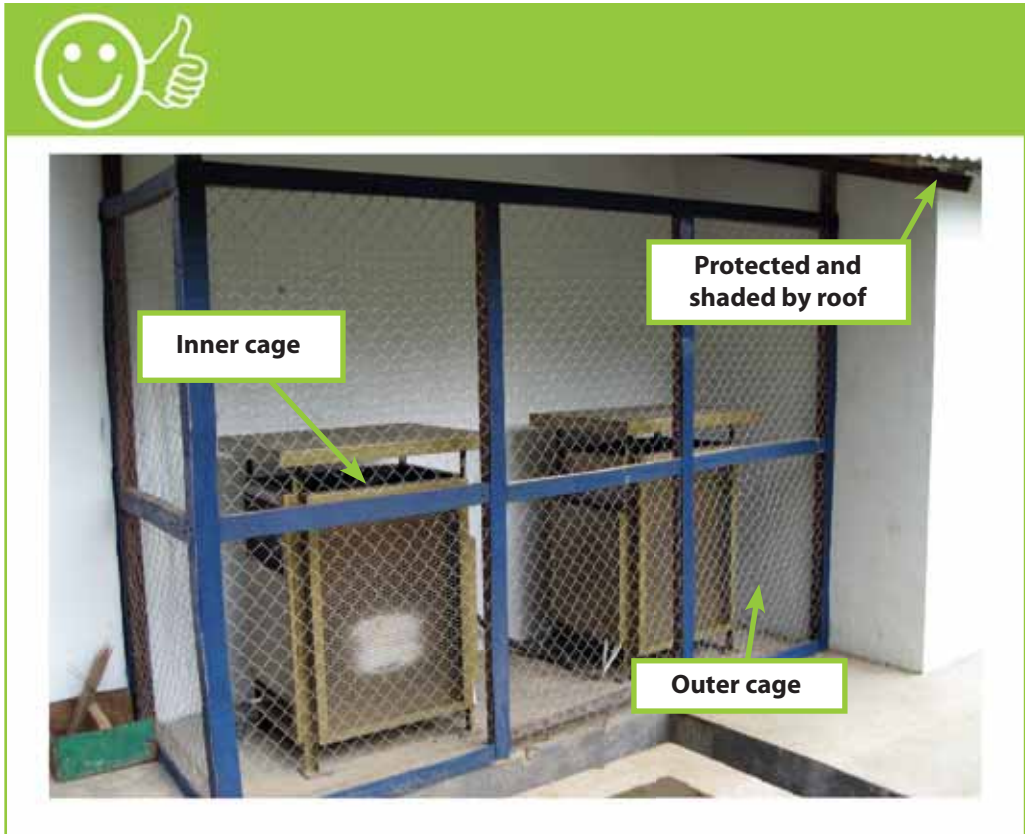
Well protected ballast at outer wall of the power house
