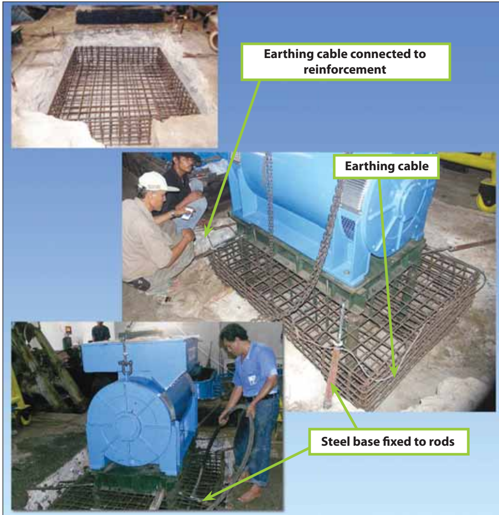
Construction details of equipment foundation
