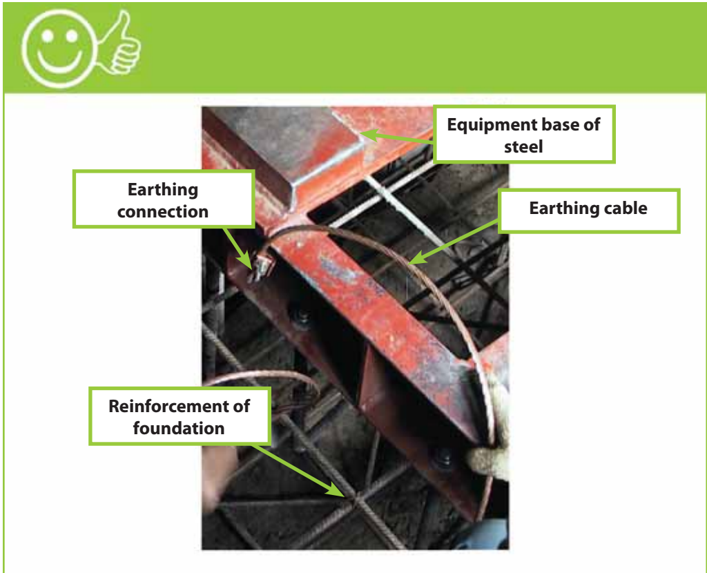
Reinforcement of foundation & steel base connected to earthing rod
