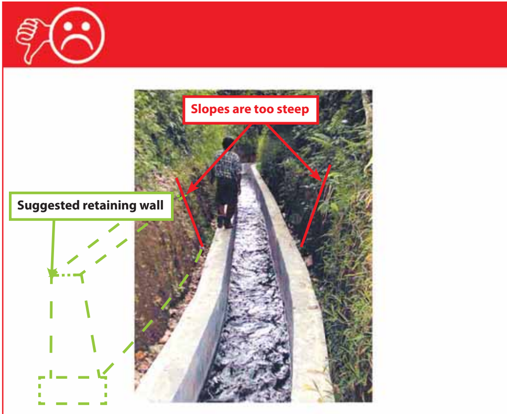
Headrace in a deep and steep cut section
