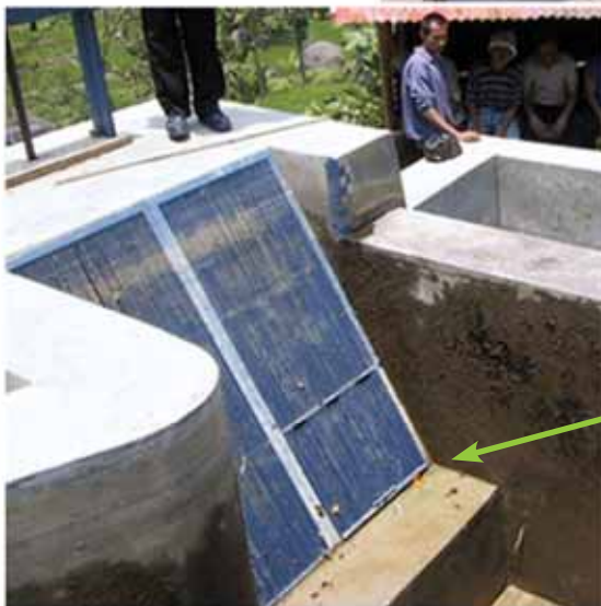
Trash rack fixed on top of a bottom sill or step, with service opening
