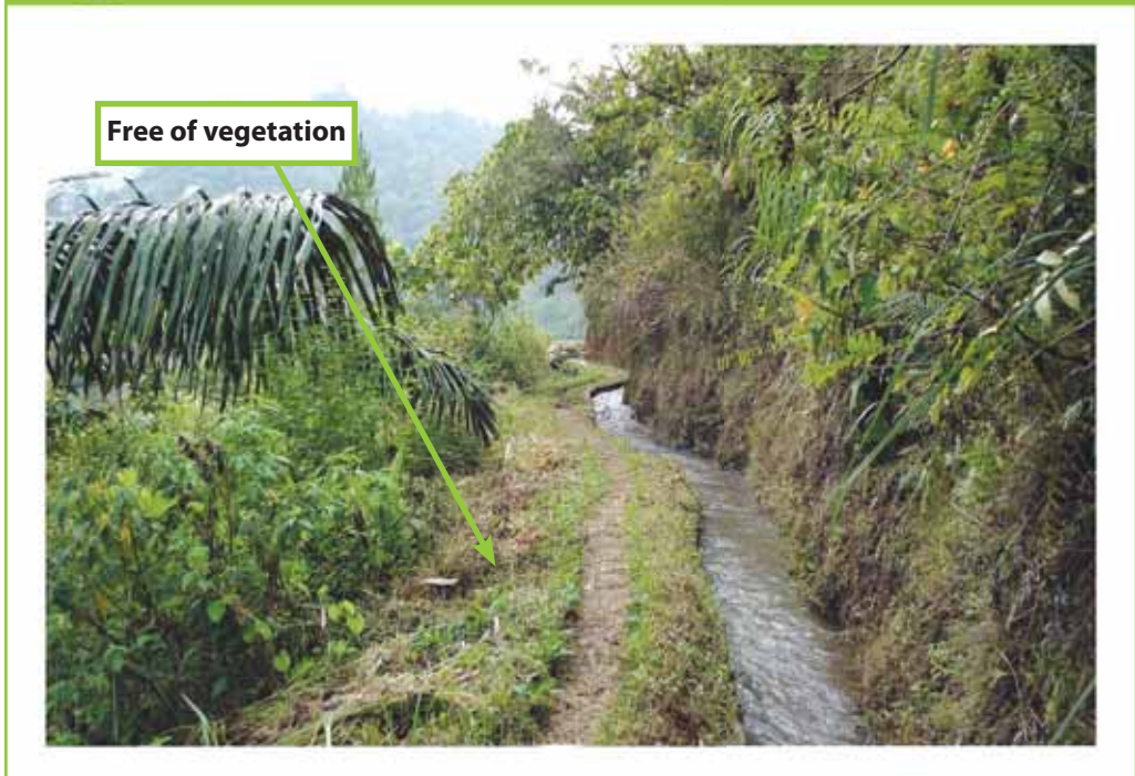
Vegetation well cut along the left bank
