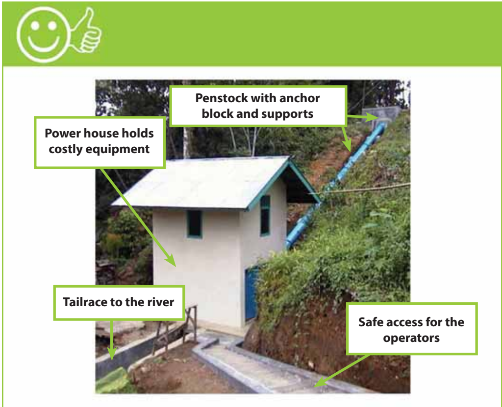
A well built and maintained power house located at a suitable place
