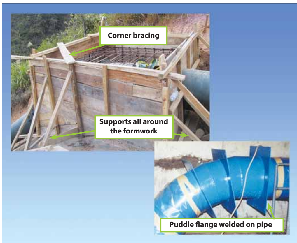
Anchor block ready for concreting
