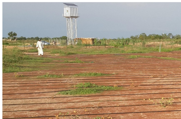
Figure 1.26: Solar powered irrigation system in Daura, Katsina
