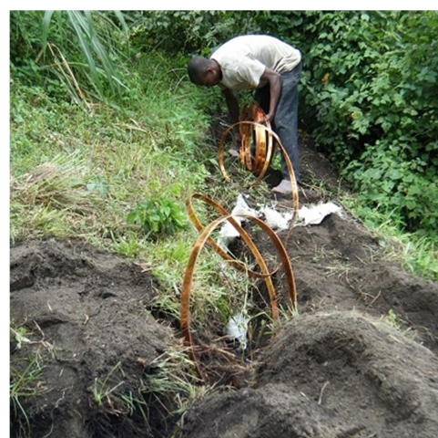
Figure 3.36: Laying a ground electrode through a solid copper band
