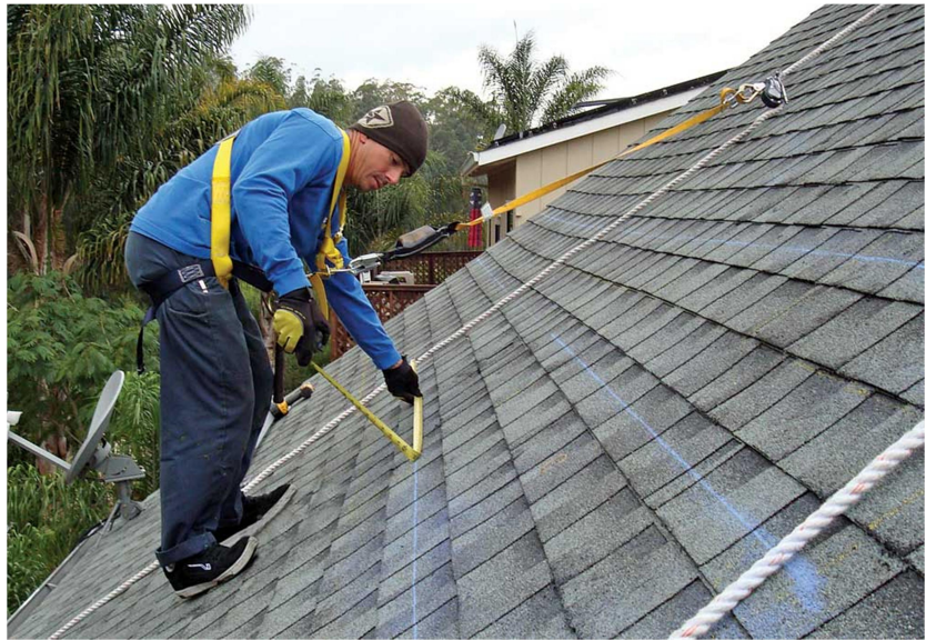
Figure 2.2: Solar PV installer in Hawaii with fall protection – Courtesy: SolarPro Magazine
