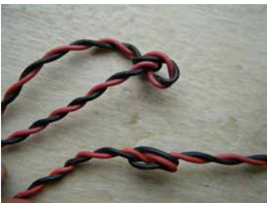
Figure 32: Freilassing cable after several months of usage.
