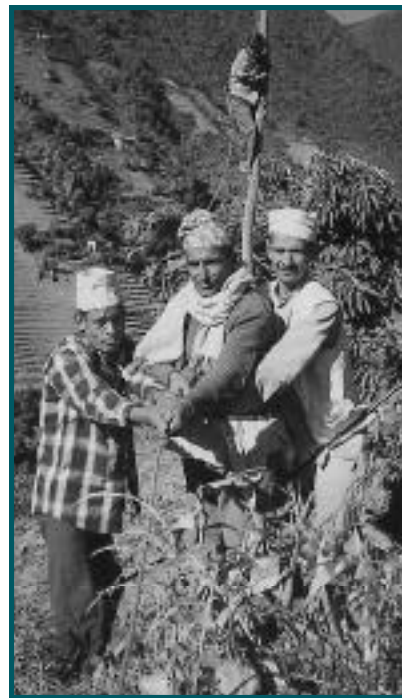
Tensioning the cable
