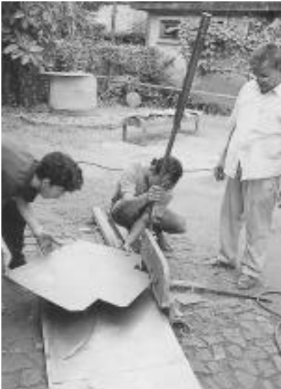
Cutting the sheet steel for the casing with a guillotine
