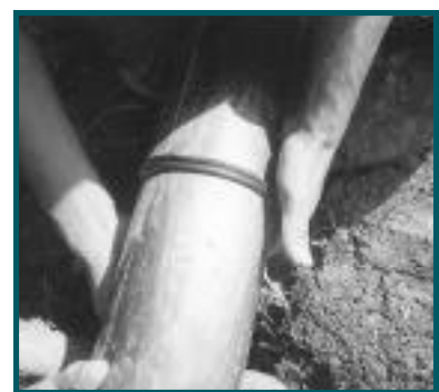
Fusion joining of pipe
