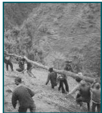
Transporting a distribution pole
